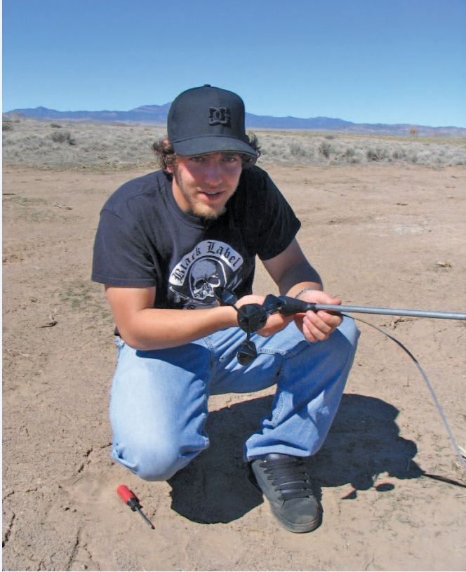
Tyson Sherwood, a student at Milford High School in Milford, Utah, affixes an anemometer to a Skystream tower for a comparison on wind speed to power output. Tyson was in the eighth grade when the first 20-meter tower was installed on teacher Andy Swapp's farm for a school project. Now Tyson is a senior who hopes to work in the renewable energy field.
